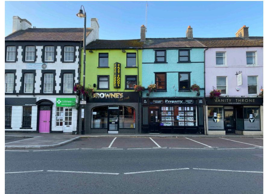
Figure 4- View of the properties on the south side of Market Square
