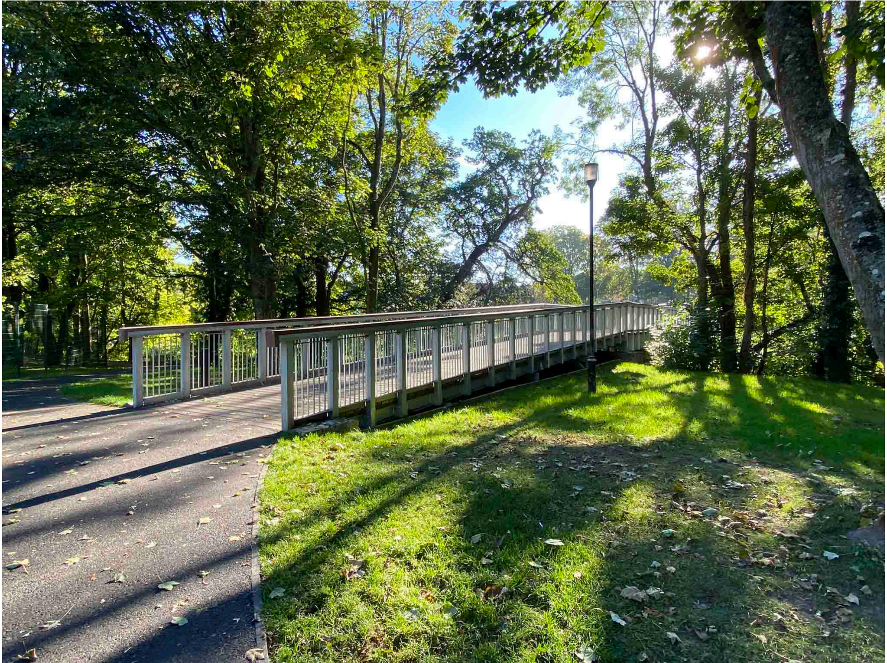
Figure 5- View of new bridge within Dromore Park leading to Banbridge Road
