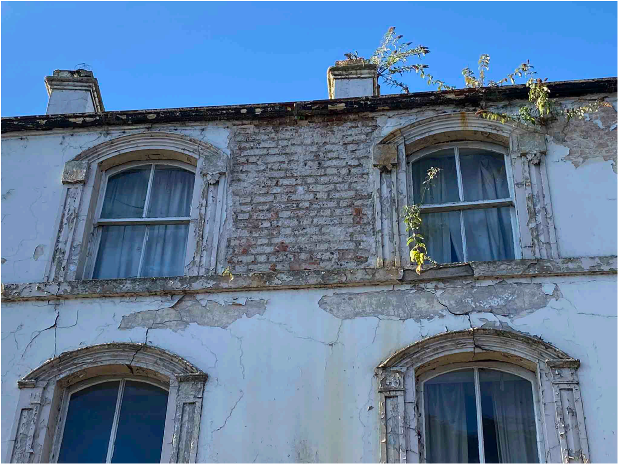
Figure 25- View of one of the buildings on Church Street
