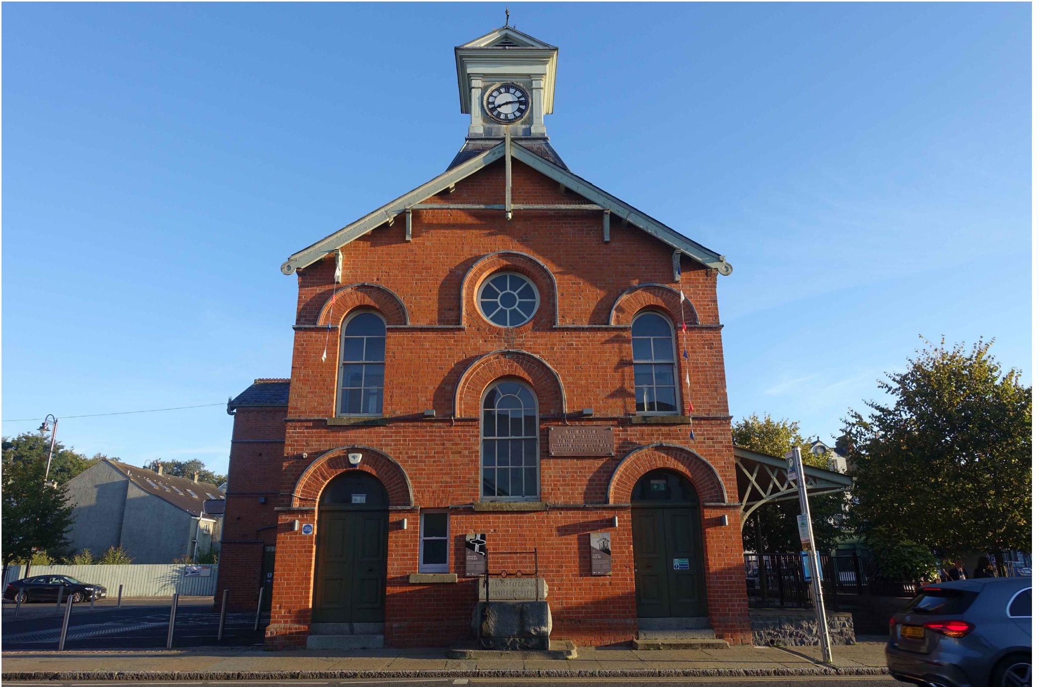
Figure 34- Early morning view of Dromore Town Hall
