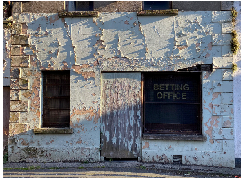
View of vacant building on Castle Street
