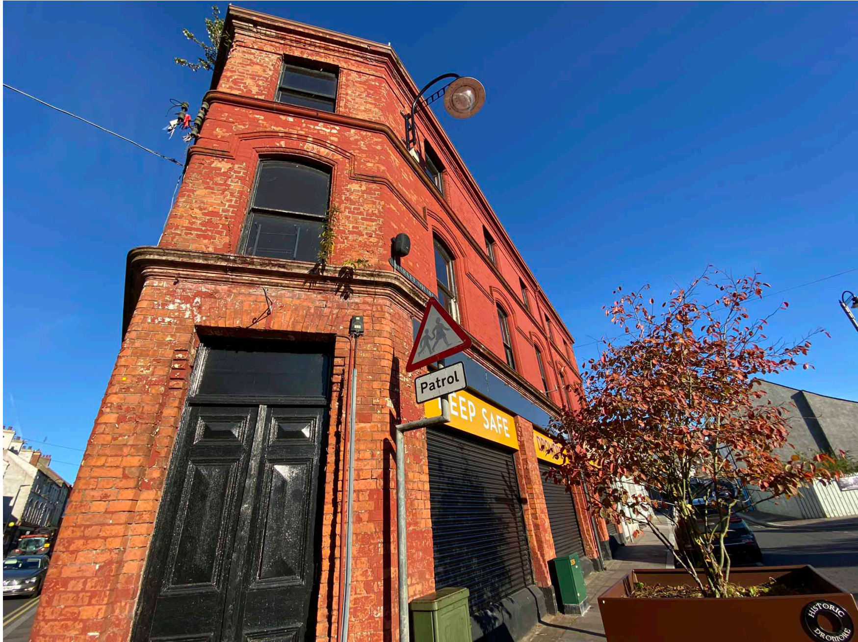
Figure 47: Corner building in Market Square
