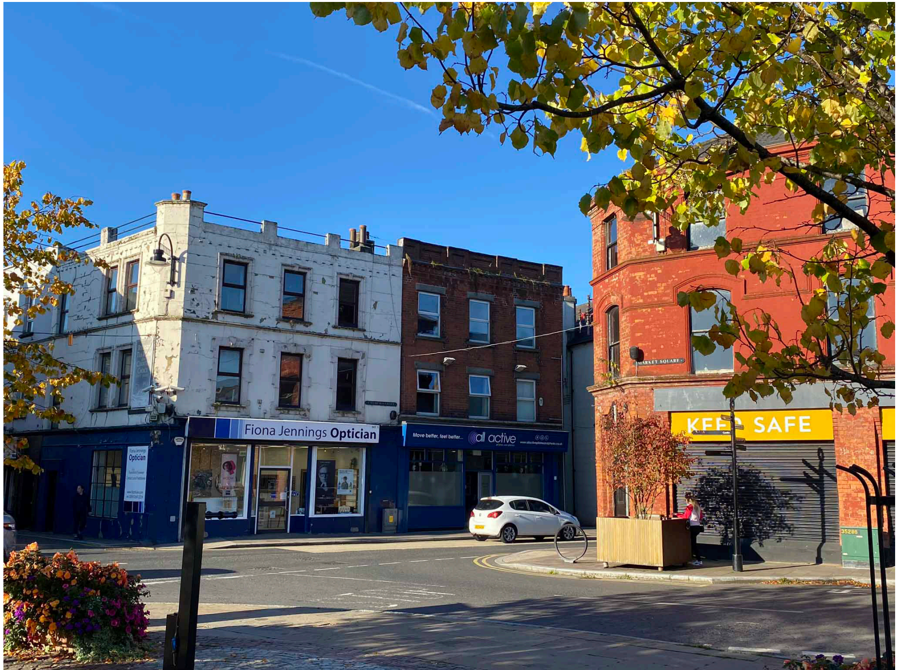
Figure 48: View of the junction at Market Square and Church Street
