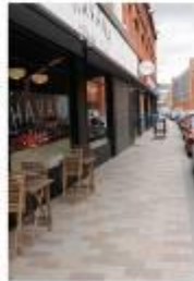
High quality natural stone paving to footways – enhancement of streetscape and opportunity to re-integrate local culture
