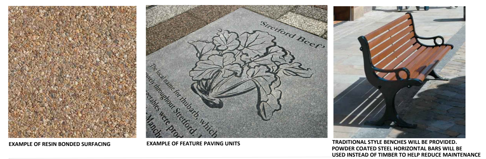
EXAMPLE OF RESIN BONDED SURFACING | EXAMPLE OF FEATURE PAVING UNITS | TRADITIONAL STYLE BENCHES WILL BE PROVIDED. POWDER COATED STEEL HORIZONTAL BARS WILL BE USED INSTEAD OF TIMBER TO HELP REDUCE MAINTENANCE
