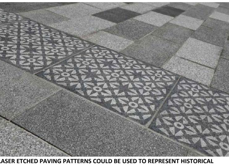
LASER ETCHED PAVING PATTERNS COULD BE USED TO REPRESENT HISTORICAL WEAVING PATTERNS OF WARINGSTOWN
